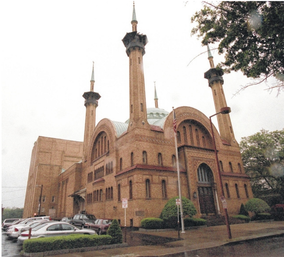
The magnificent Irem Temple—repairs are progressing
