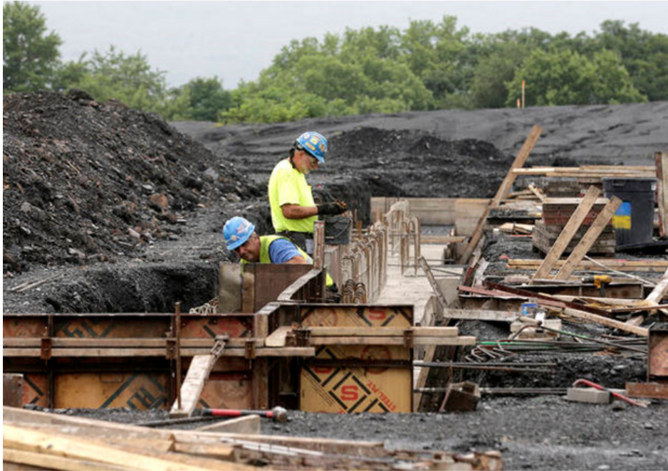
Contractors work on part of the foundation for the new Wilkes-Barre Area consolidated high school Monday foundation Bill Tarutis | For Times Leader
