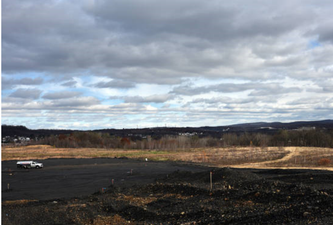
The truck in the distance sits roughly to the right of what is to be the main entrance of Wilkes-Barre Area’s new consolidated high school. - Aimee Dilger | Times Leader
