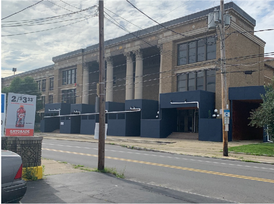
Meyers as of July 2019 with attractive board provided gutter add-ons. Picture by Kate Kelly
