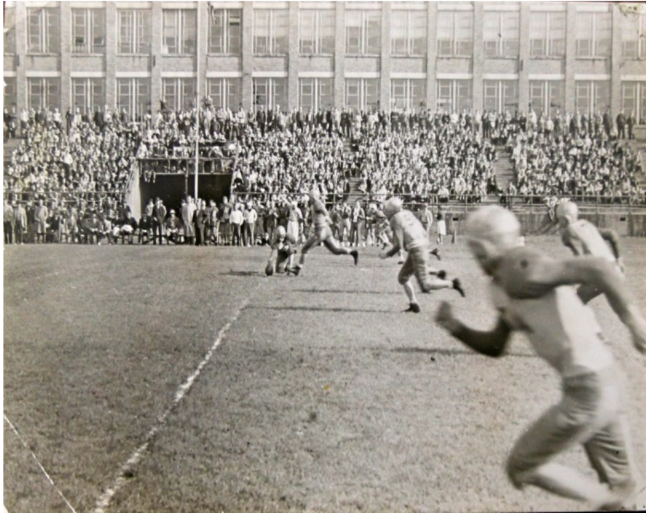
Concrete Bleachers hugged Meyers High in the stadium's Glory Days. They are now gone.
