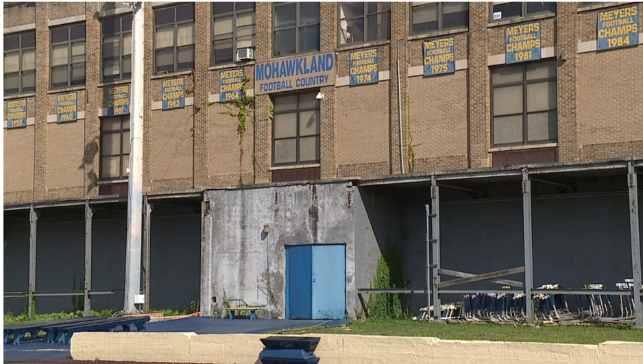
High School Stadium in Wilkes-Barre Closed for Repairs
